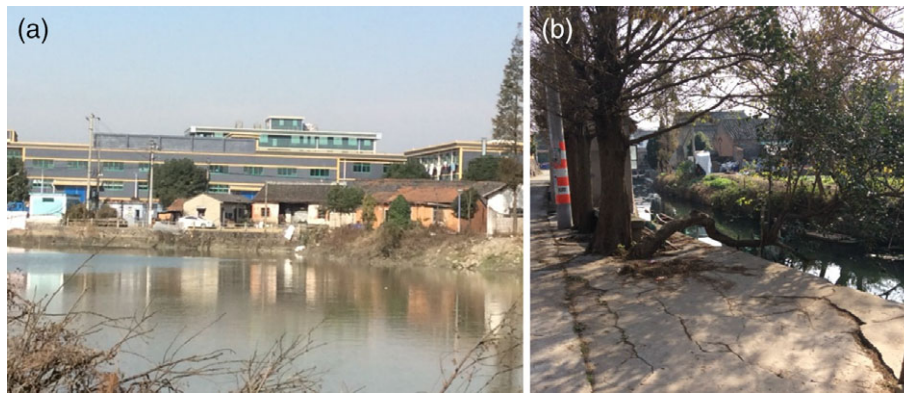
FIGURE 3 Contrast between an embankment made of artificial and natural materials. (a) Contrasting channel bank treatments adjacent to Wujingqi: The section on the left has been reinforced using concrete and masonry and can easily support modern buildings and a roadway, while the section to the right, which is still formed in soil reinforced by trees and shrubs, can only support an old-style of building. (b) Contrasting bank treatments along a channel connecting a water gate on the Nantang River to the Fenghua River at TangJiaShi Yan: The near bank is covered by concrete that is cracked and failing. The opposite bank is stabilised by natural vegetation with little or no artificial reinforcement and probably resembles conditions that pertained prior to the availability of artificial materials such as concrete (both photographs by the authors, December 6, 2014)
