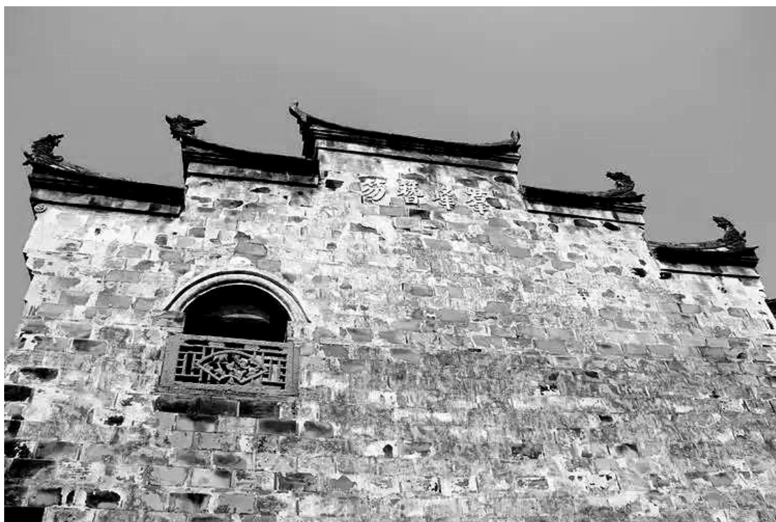
Figure 3.16 The Horse head walls in QunFengZanHu House
