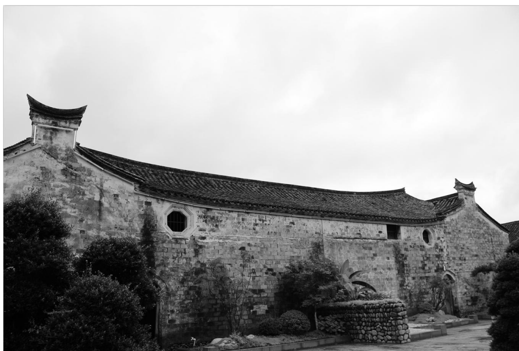
Figure 3.17 The back walls in QunFengZanHu House
