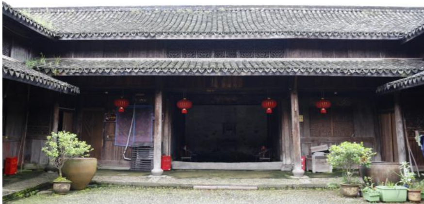
Figure 2.13 Courtyard and open hall (Photographed by the author 2021)
