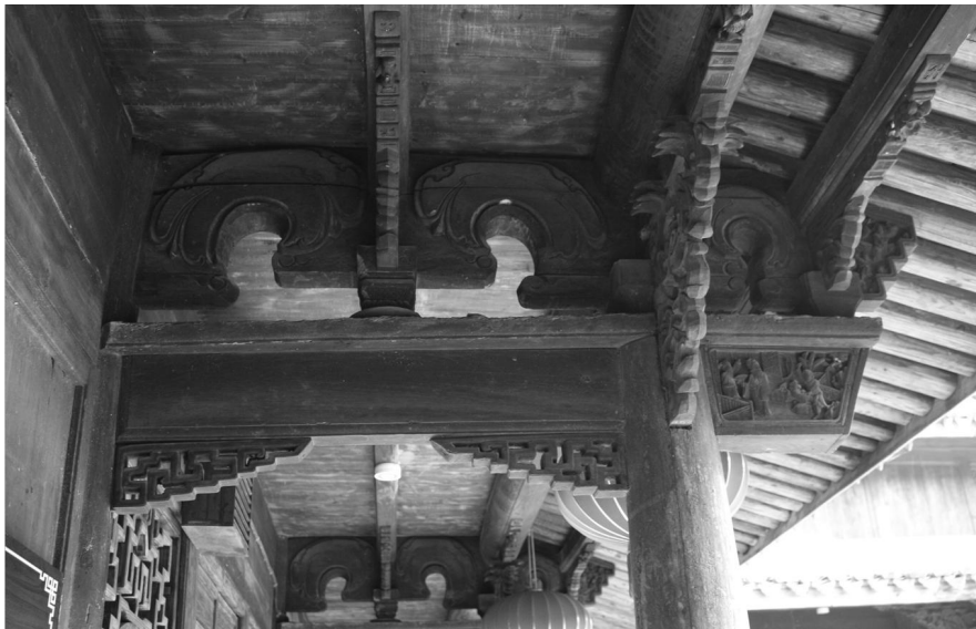
Figure 3.22 The double span crescent beams
