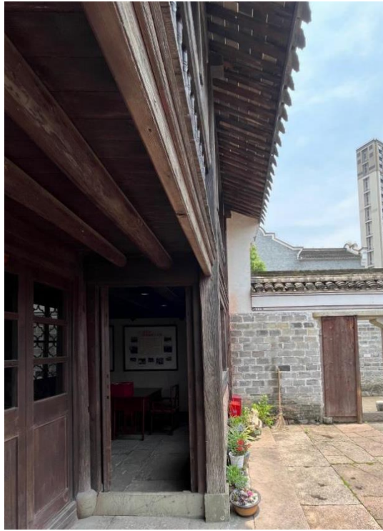
Figure 4-6. The eave of Yan's former residence.
