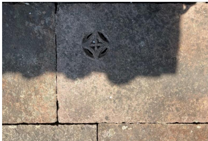
Figure 4-12. The drainage hole.
