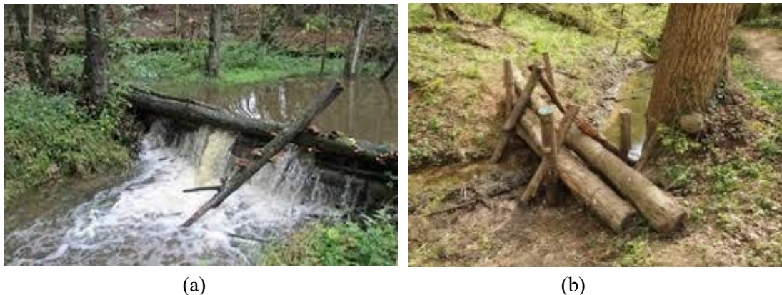
Figure 48 Leaky wooden dams (a) and (b). (Yunfei Qi)
