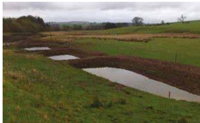
Figure 45 A series of constructed sediment traps. (Yunfei Qi)
