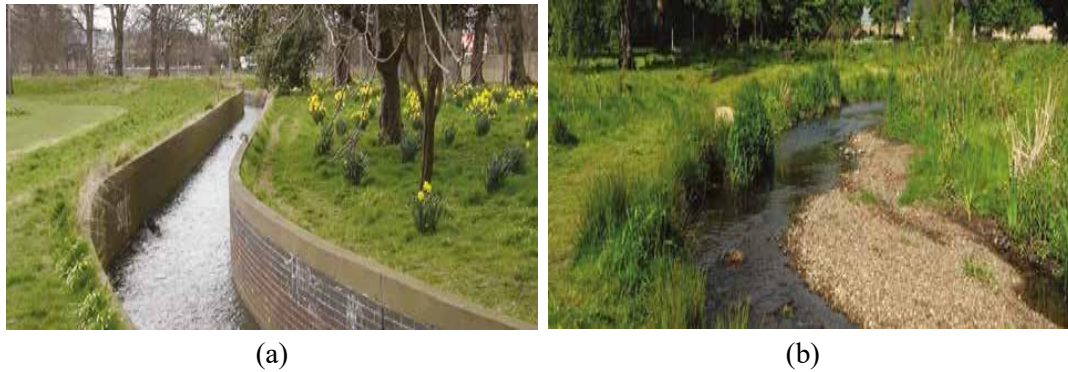
Figure 47 Removing an artificially raised bank (a) and replacing the concrete channel with NFM measures (b). (Yunfei Qi)
